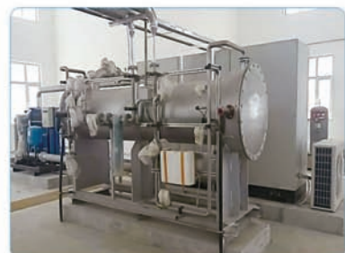
Hubei Wuhan Municipal Water Supply Project
