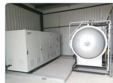
Anhui Mingguang Water Treatment Plant Project
