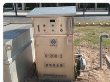
Jiangsu Huai'an Food Factory Project
