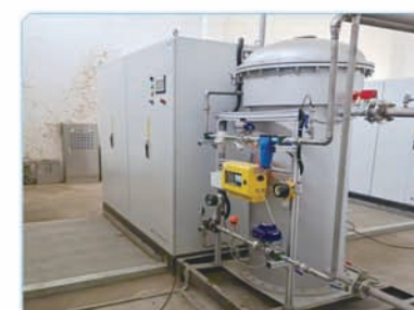
Shandong Binzhou Sewage Treatment Plant Project
